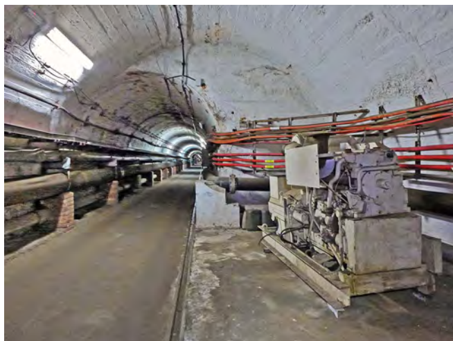
Admiralty Tunnel: a short bay section just inside the Dockyard portal
